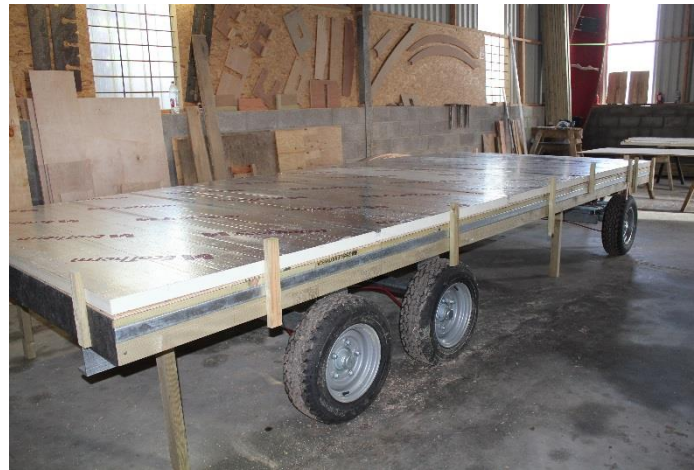
Solid floor construction
