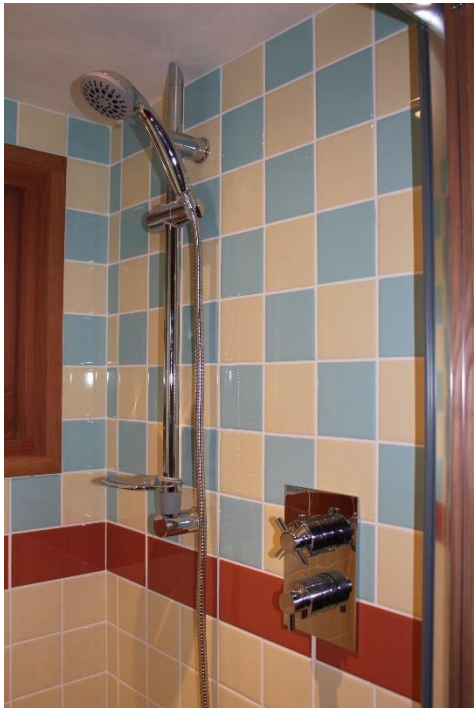
Fully tiled & plumbed shower
