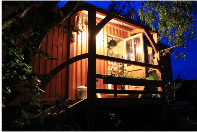
Timber frame veranda
