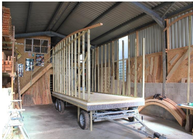
Curved roof shape & frame
