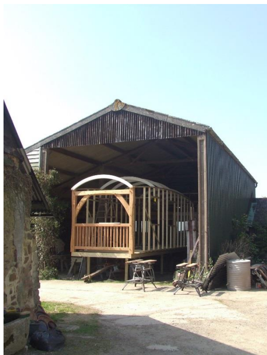
Laminate ribs and frame
